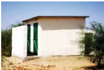
Top: New pre-school shelter under construction
